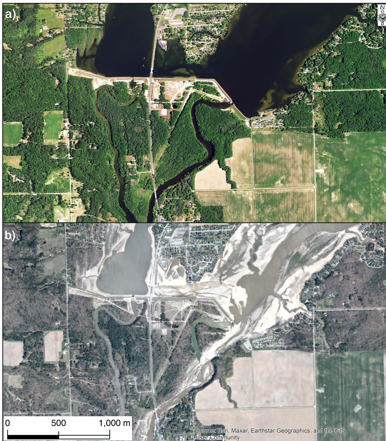
Figure 3. (a) Pre-failure and (b) post-failure imagery of the Edenville Dam. The approximate failure location where the depression was observed is shown in red. (Pre-failure imagery: NAIP image; post-failure imagery: ArcGIS world imagery.)
